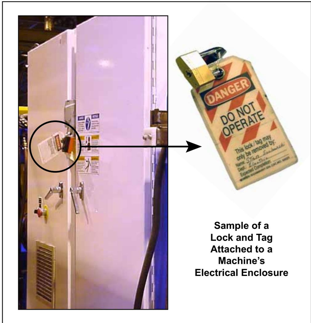
**When Working on a Machine Inside the Machine's Main Electrical Enclosure or in the Electrical Transmission Line to the Machine**
